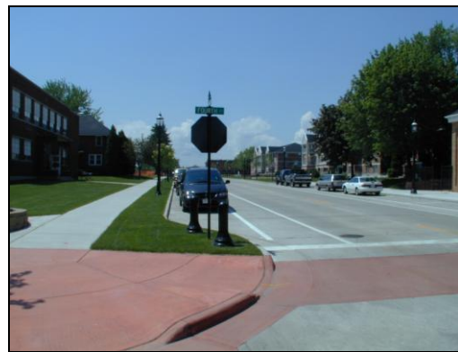
Curb extension along Grant Street in De Pere
