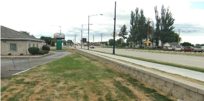
Retaining wall minimizes impacts. Similar approach could be used in front of wetlands near Optimist Park.
