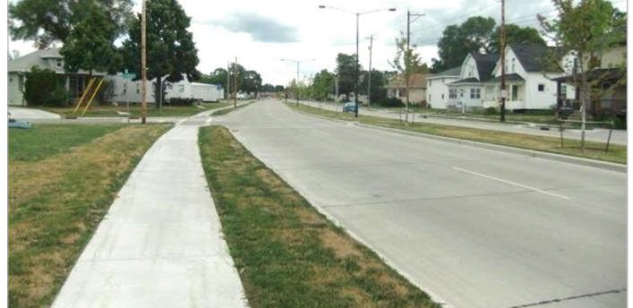
Completed Velp Avenue with added sidewalk and storm sewer throughout.
