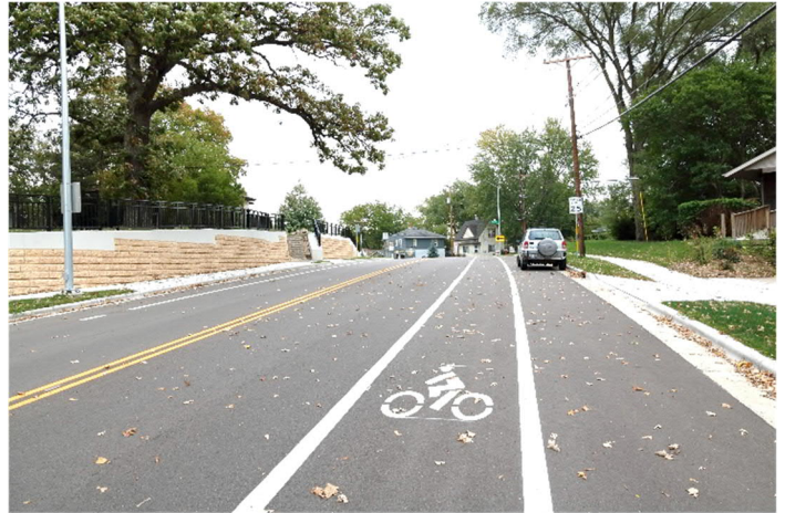
Reconstructed Buckeye Road using retaining walls in select locations to avoid impacts to mature trees. Similar but shorter walls may be proposed for Libal Street for similar reasons.
